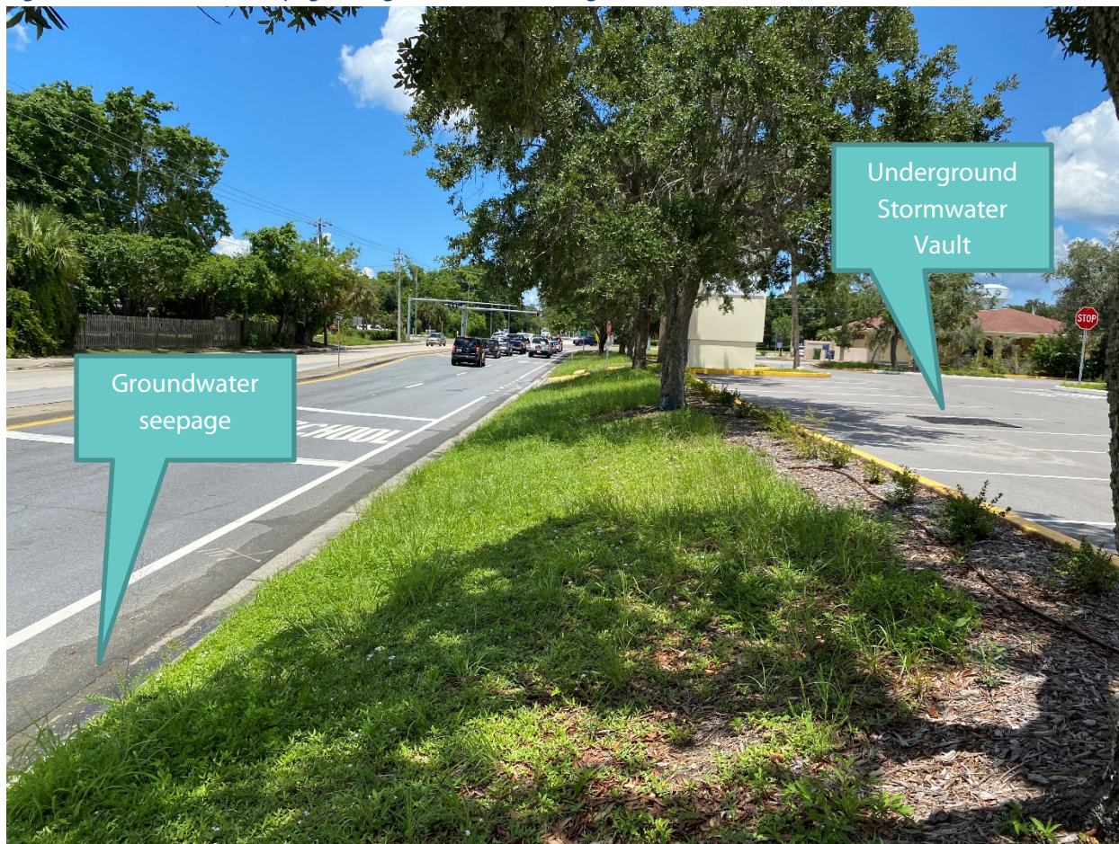
Figure 15: Groundwater Seepage along 75th Street (looking north)
