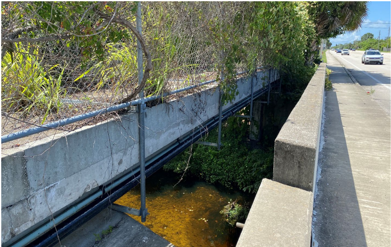
Figure 19: Utility bridge (looking south)
