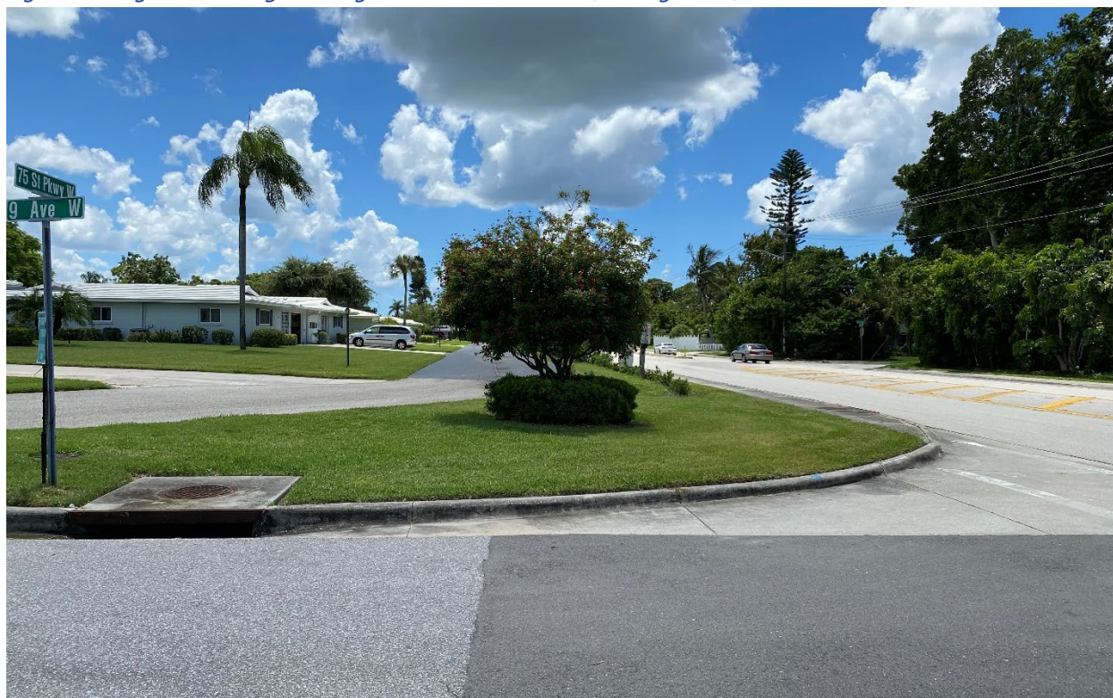
Figure 11: Vegetation in Sight Triangle of 9th Avenue West (looking south)
