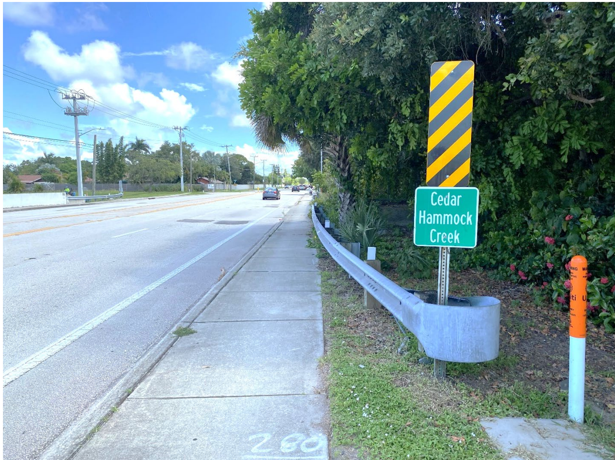
Figure 22: Bridge over Cedar Hammock Creek (looking north)
