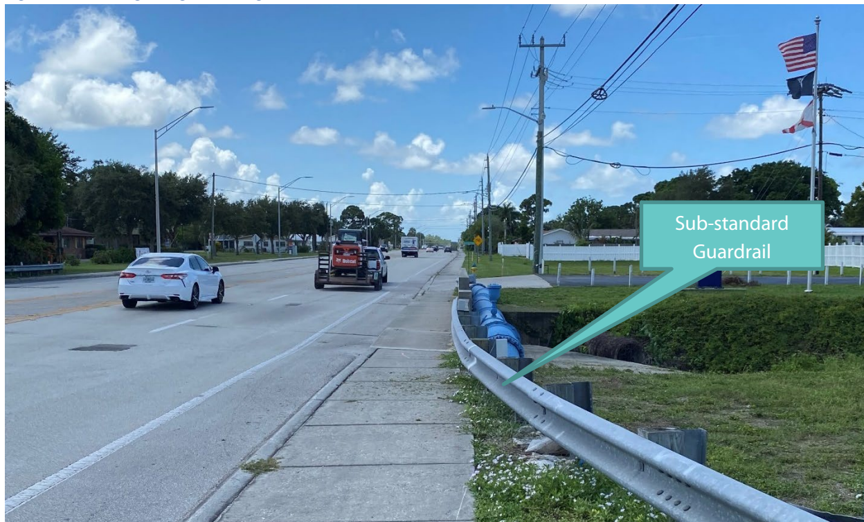
Figure 38: Existing Bridge (looking south)
